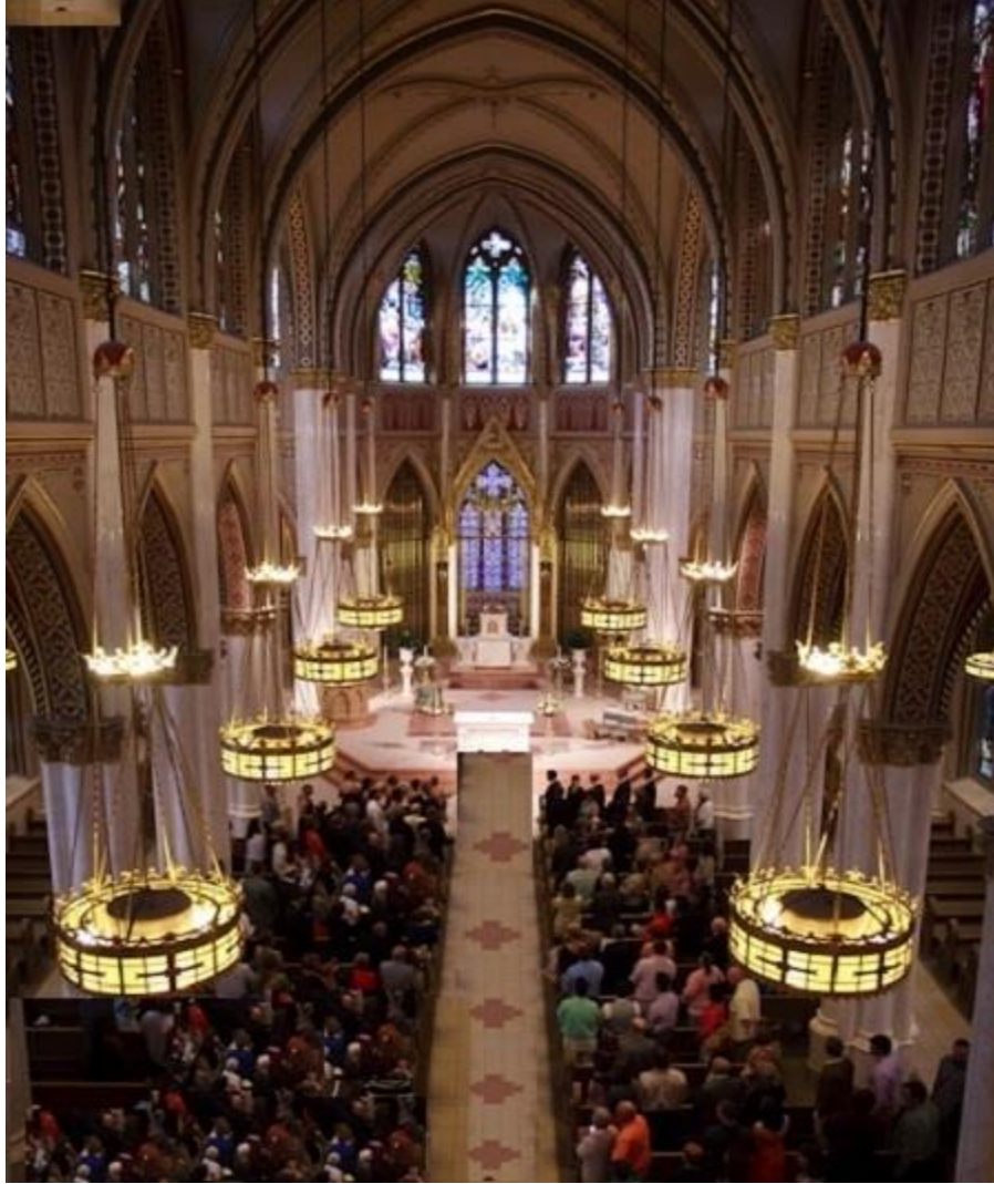
Cathedral of Saint Helena, Helena, Mont. Construction 1908-1914. In 1913, Thomas Cruse donated $3,139,194.00 (current value of money) to the Diocese of Helena to finish and furnish the interior of the Cathedral. His total donation was $5,674,960.00 (current value of money). Photo courtesy Megan Lane Photography, Helena, Mont. Megan Lane Photography dot com.
