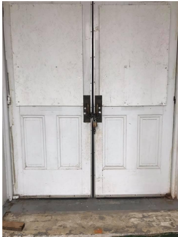
Figure 8. Bryce hospital doors. A padlock and chains lock the front doors to the main building of Bryce Hospital currently under renovation. February 14, 2019.
