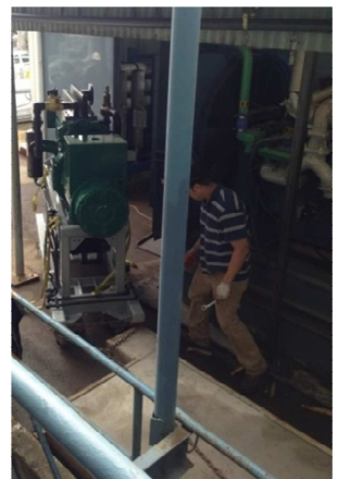
Figure 7-2. Full-scale PSE being moved in on the concrete foundation during installation.
