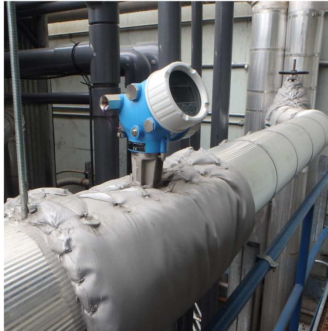
Figure 7-4. Installation of the flow meter.
