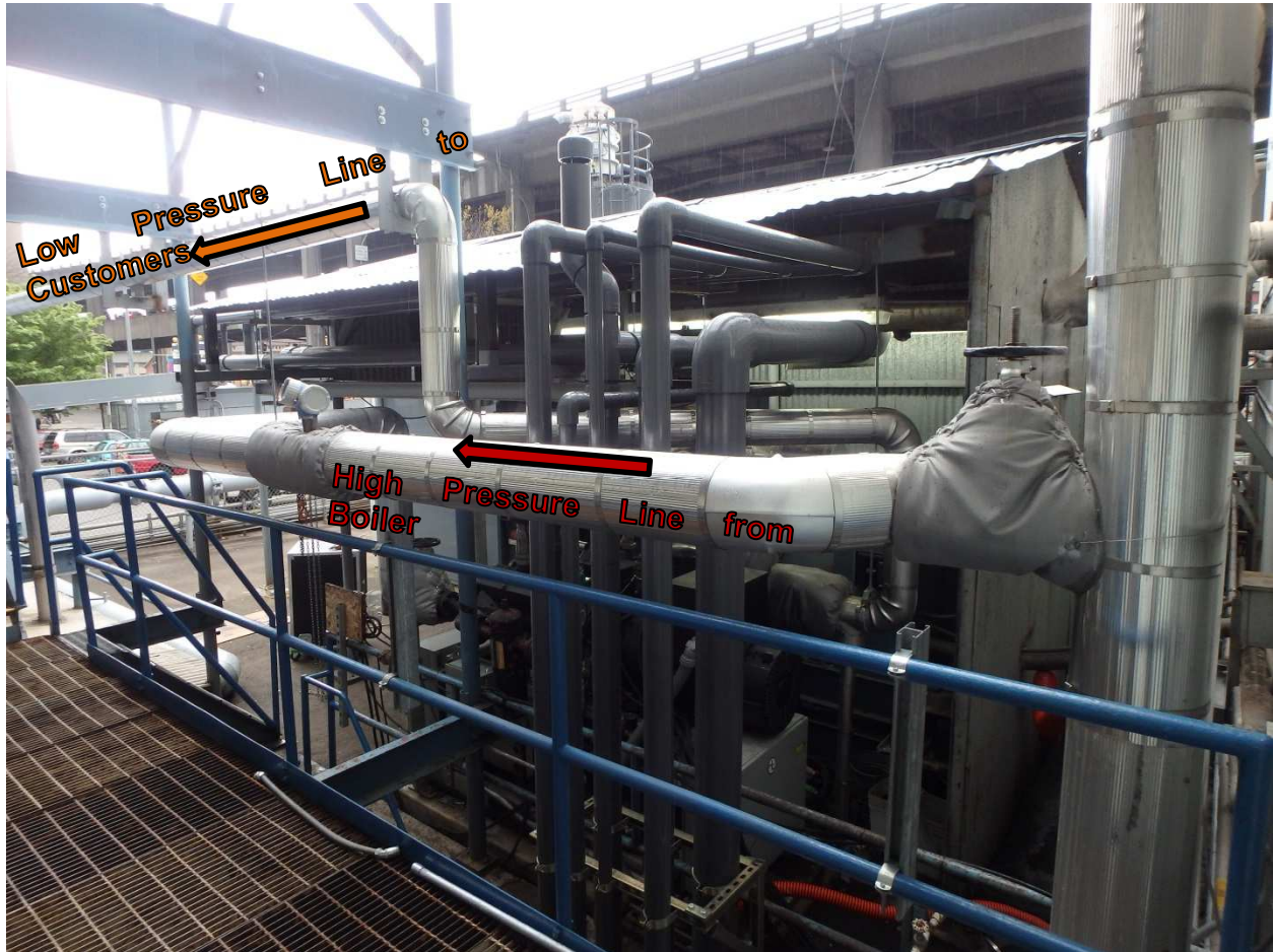
Figure 7-3. Final installation of the PSE at Enwave Seattle.
