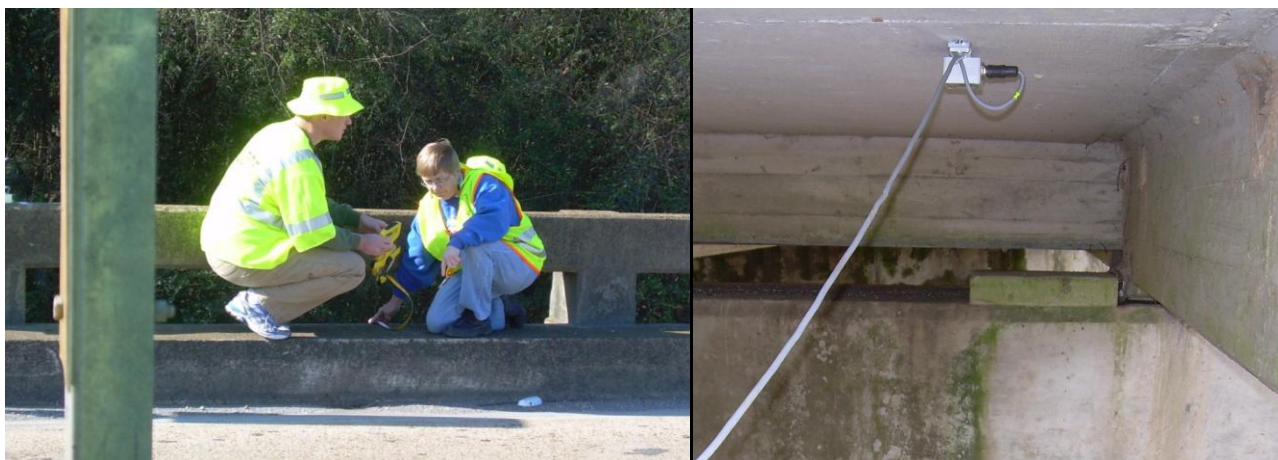
Figure 3.13 Measuring Distance to wheel path/Longitudinal axle detector sensor
