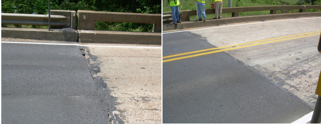
Figure 3.5 Photo of two expansion joints
