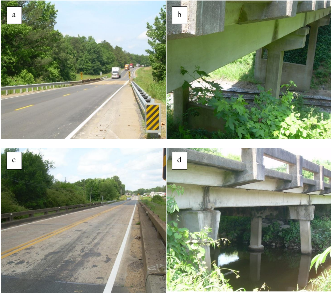
Figure 3.6 Photos of bridge 1 (a & b) and bridge 2 (c & d)
